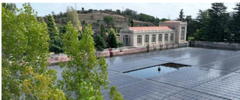
Picture 3. Floating photovoltaic solar plant in Torrelaguna (Madrid)
